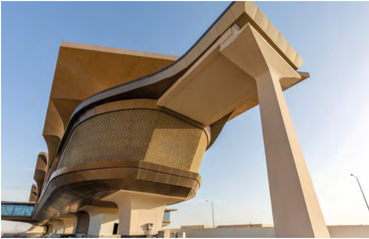
▲ Doha Metro Elevated Stations Architectural Finishes (Qatar)
